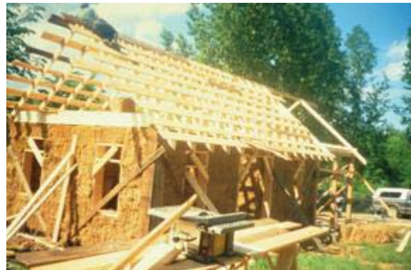
Building with straw bales.
