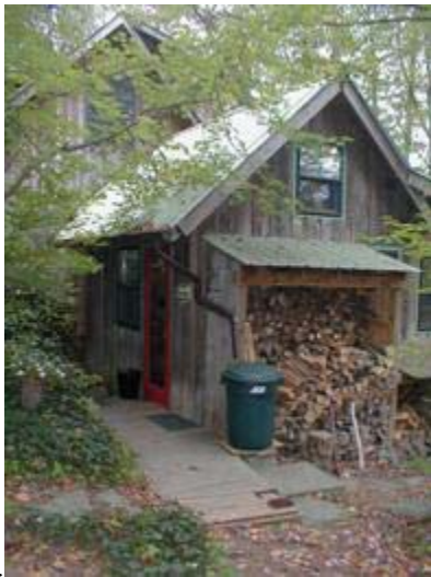
Water catchment System
